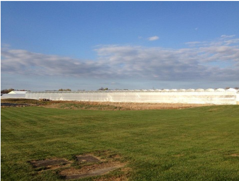
Image 2: Greenhouse Construction Site in Belvidere, New Jersey
