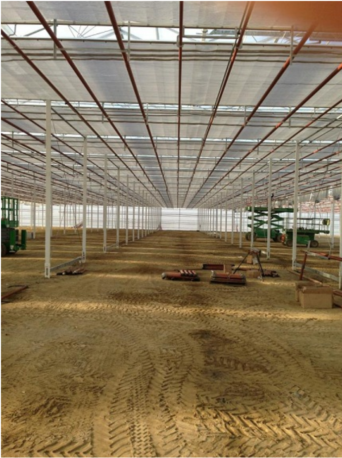
Image 1: Greenhouse Construction Site in Belvidere, New Jersey
