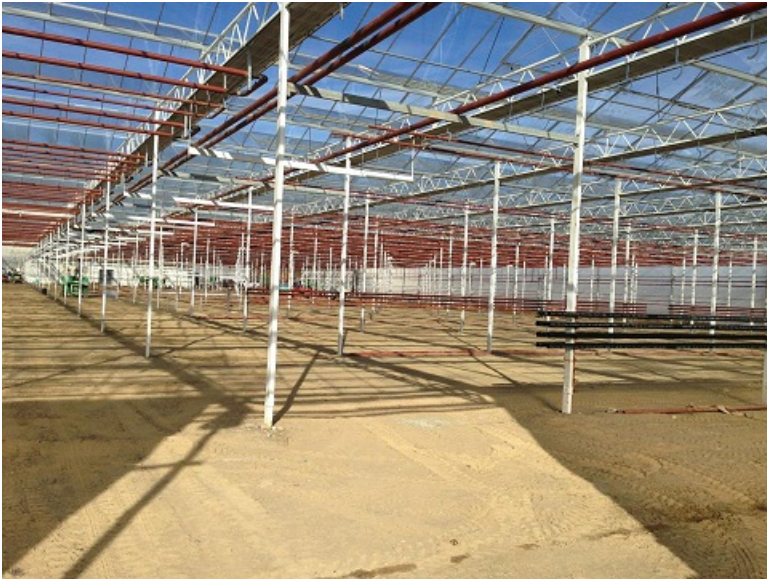
Image 3: Greenhouse Construction Site in Belvidere, New Jersey
