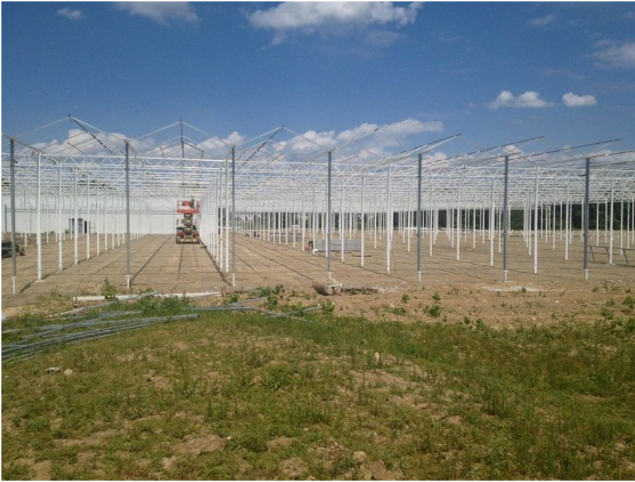
Image 3: Greenhouse Construction Site in Belvidere, New Jersey
