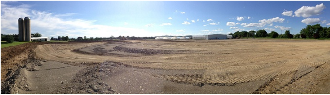
Image 1: Greenhouse Construction Site in Belvidere, New Jersey
