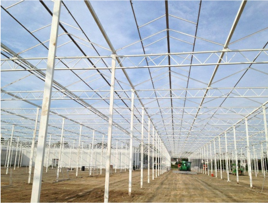
Image 2: Greenhouse Construction Site in Belvidere, New Jersey
